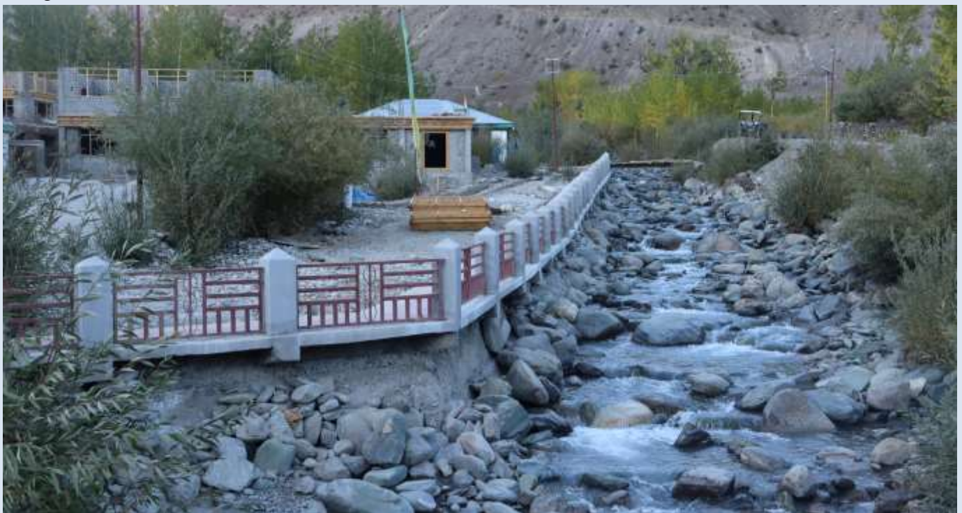
Field Photograph of Flood Prone Nallah
